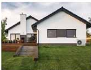
Air Source Heating
